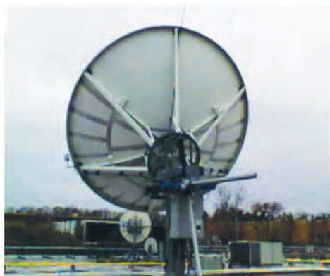
Figure 1: Antenna Rear – Surface / Pad Heated Anti-icing
